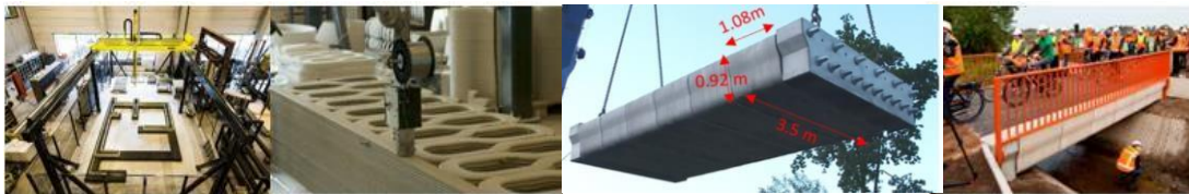
Figure 1. The case study bridge and printing process at TU/e (Bos et al. 2017)
