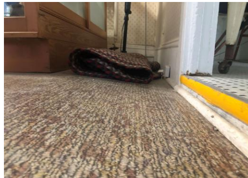
Figure 4. Typical floor conditions
