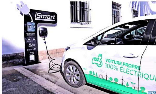
Fig. 4. Chargers in Morocco inaugurate by IRISEN, charging power of 20 kW
