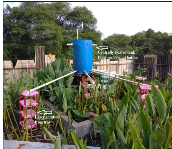
Fig. 1(b) Feeding cum aeration system of VFCW
