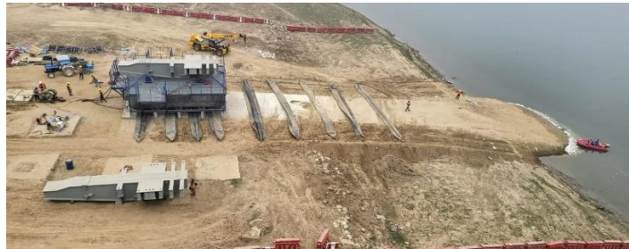
d) Assembly Area on Naini river Bank
