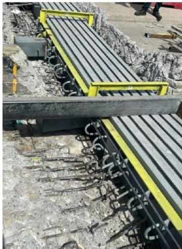
i) Setup of new expansion joint
