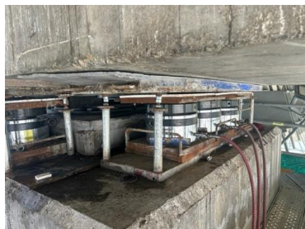
h) Bearing replacement
