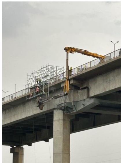
g) negative scaffolding erection
