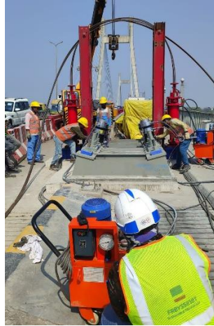
f) Upper deck beam connection
