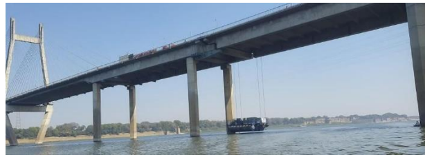
a) Naini Bridge
