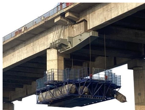
e) Lifting down of platform
