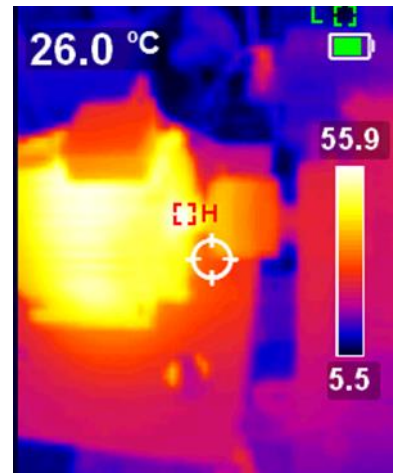
4. Figure. Asynchronous motor connected to a load machine (side view).
